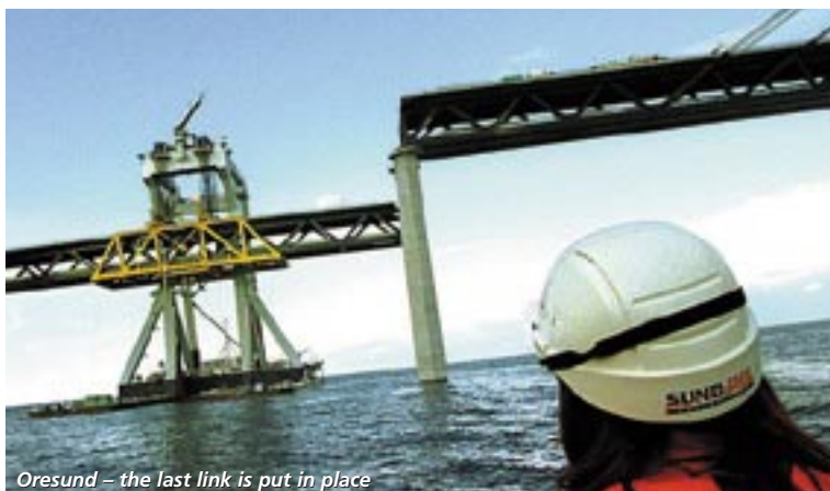
Öresund – the last link is put in place
